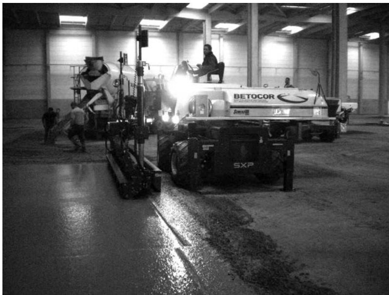
Figure 34.13 Steel-frc floor installation. (Supplied by J. Greenhalgh, Bekaert Ltd, UK, www.bekaert.com )
