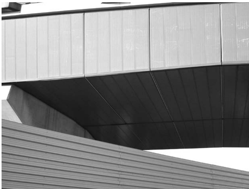
Figure 34.9 Photograph of the enclosure on the approach span of the Dartford River (or QE2) Bridge where it passes over the Channel Tunnel Rail Link (before the train rails were laid). (Courtesy of AECON.)
