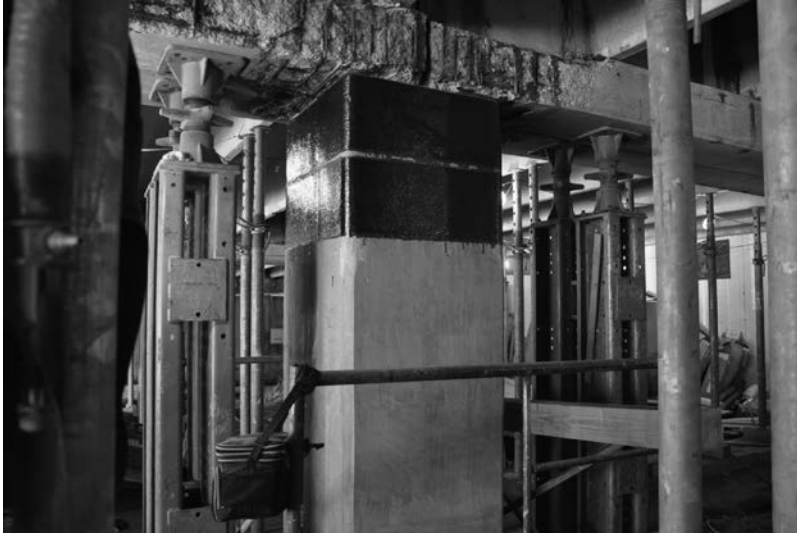
Figure 34.6 Wrapping of a degraded RC column top with CFRP. (Reproduced courtesy of American Concrete Institute (Georgia Chapter), http://aci-ga.org )
