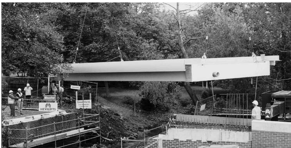
Figure 34.1 Structural deck of the West Mill Bridge (Oxfordshire, UK) being lifted into position. (Photo reproduced by courtesy of Fibreline Composites, https://fiberline.com/ )
