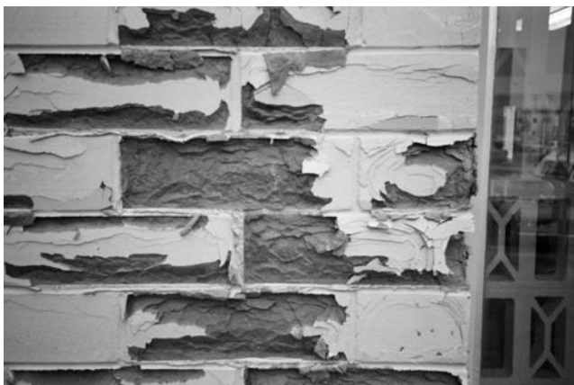
Figure 50.4 Erosion due to frost attack.
