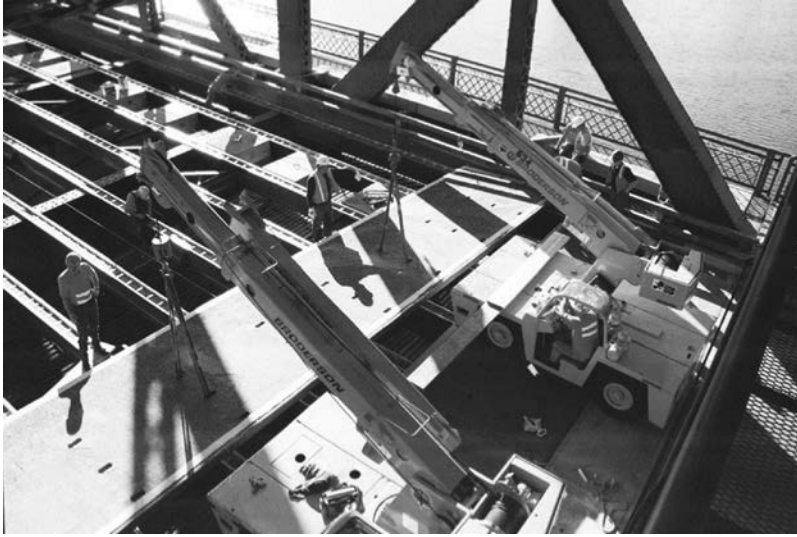
Figure 34.2 Frp deck panels being installed using fork-lift trucks on the Broadway Bridge, Portland, OR. (From Sams M, 2005, Broadway bridge case study: Bridge deck application of fiber-reinforced polymer, in Transportation Research Record: Journal of the Transportation Research Board , CD-11-5, Figure 5, p 177, Transportation Research Board of the National Academies, Washington, DC, pp 175–178, reproduced with permission of the Transportation Research Board.)
