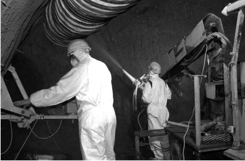
Figure 34.12 Tunnel lining (steel-frc) spraying equipment. Note the segmental extendable arm (top right, in partially retracted position) and computer control systems for laser guidance and monitoring (left). (Reproduced from the presentation accompanying Eddie C M and Neumann C, 2004, Development of the LaserShell method of tunnelling, in Proceedings of the North American Tunnelling Conference , Atlanta, GA, eds. O Levent and O Ozdemir, Taylor & Francis, London, UK, by kind permission of the authors and Morgan Est Ltd/Beton-und Monierbau.)
