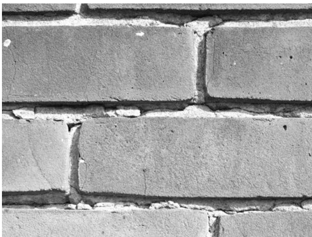
Figure 50.2 Sulphate attack of mortar.
