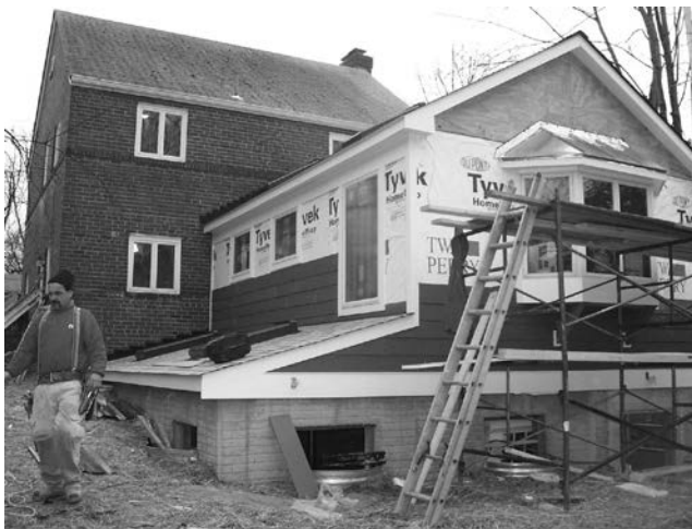
Figure 34.14 Natural-frc sidings being installed. (Photo by Mark Zimmerman, US, 2007, reproduced from flickr.com/photos/pdz_house under Attribution 2.0 Generic License [see creativecommons.org for license details].)
