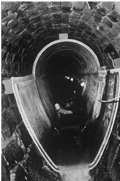
Figure 34.15 Glass-frc sewer linings in London, UK. (Reproduced from Banthia N et al., 2012, Fiber-reinforced concrete in precast concrete applications: Research leads to innovative products, PCI J , Summer, 33–46, http://www.pci.org/publications/pci_journal/2012/summer/fiber-reinforced_concrete_in_precast_concrete_applications_research_leads_to_innovative_products/ (accessed July 2016), with kind permission from the author.)
