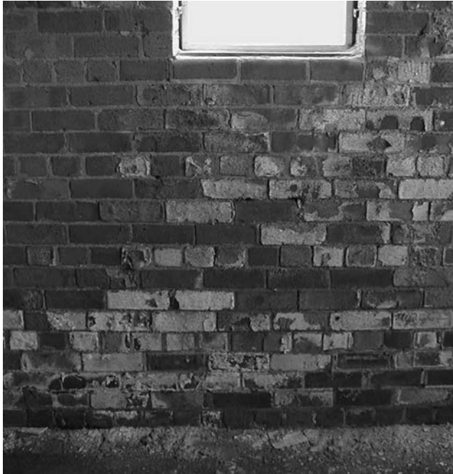
Figure 50.5 Salt crystallisation damage to masonry together with associated efflorescence.
