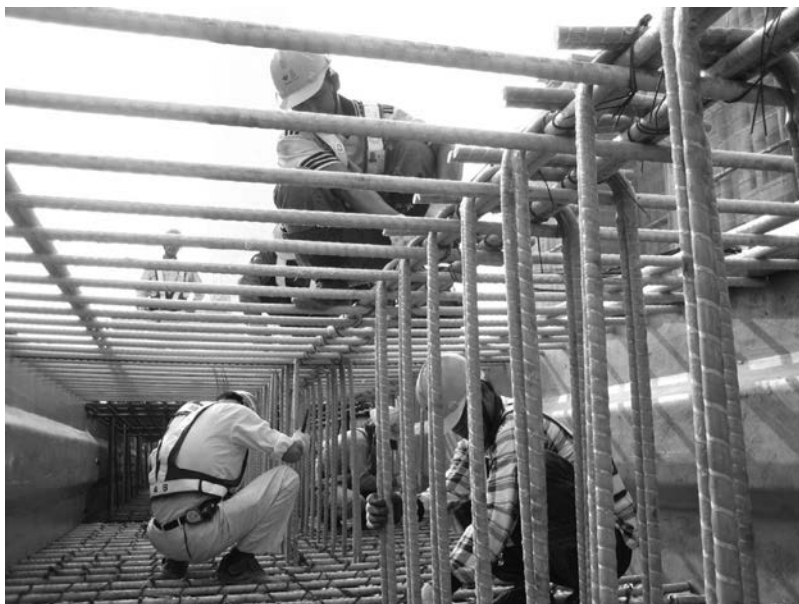
Figure 34.7 Frp rebars. (Reprinted with permission from ACMA and the Transportation Structures Council, http://www.acmanet.org )
